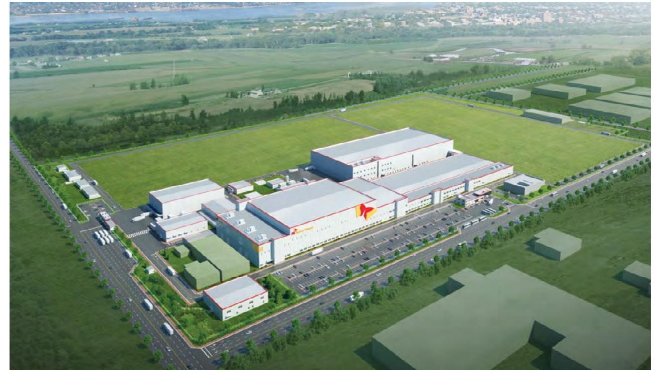
Establishing battery production facilities in Hungary (Expected to be completed by 2020)
