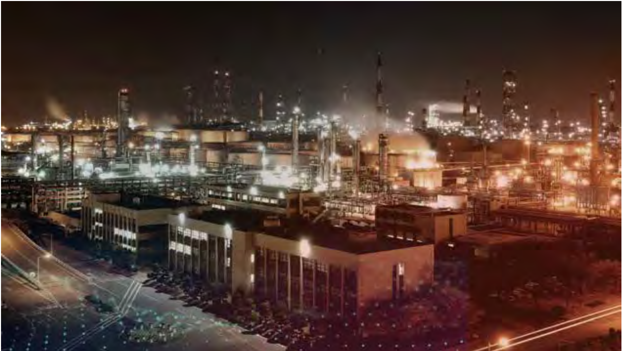
Front view of the plant from the main building of SK energy Ulsan Complex
