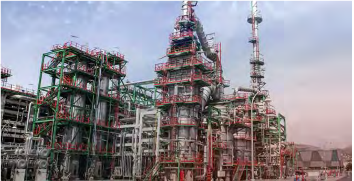
LBO Plant of ILBOC Spain(joint company of SK lubricants and Repsol)
