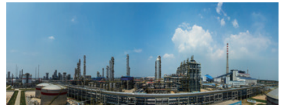
A complete view of Wuhan plant in China.
