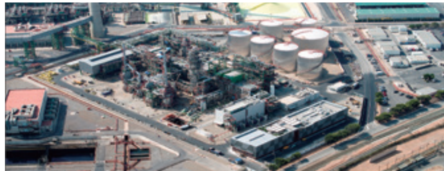
A production plant for lube base oil in Cartagena, Spain.
