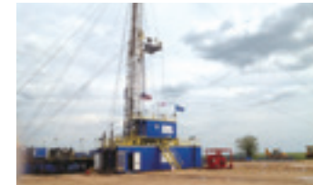
A drilling site for developing unconventional resources in Oklahoma, US.
