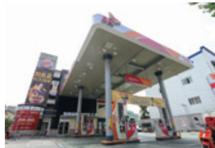
A multi-purpose gas station with self-service in Sangjin, Daegu.
